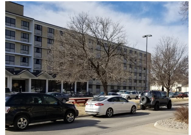
Street parking in front of McMindes Hall
